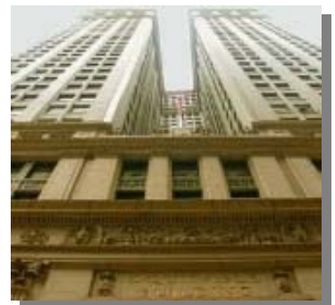
The first zoning regulations were adopted due to the reaction from the construction of the Equitable Building in New York City. Photo: http://www.earthdocumentary.com/equitable_building_new_york_city.htm
