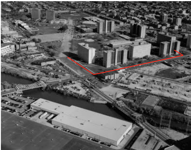
The Cabrini Green housing project (located in Chicago, Illinois and marked within red border) was separated from the rest of the City by a large freeway. Photo: http://reference.findtarget.com/search/urban%20renewal/ .
